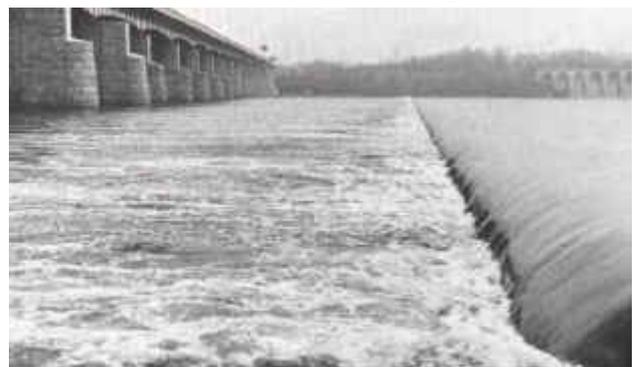
around such hazards. In order to successfully "run " the dam, your boat must clear the downstream backwash and boil and enter the outwash area. As the water level rises, the boil and backwash area move downstream and the potential of becoming trapped in the drowning machine becomes a sure thing.
